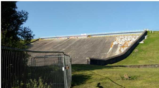
Rockfill on the right side the Toddbrook Spillway
