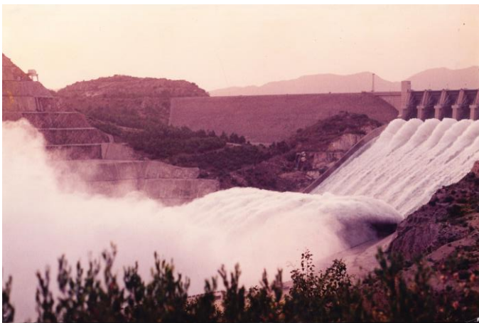
Tarbela Dam's main spillway
