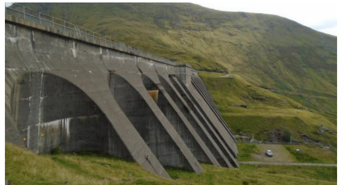
Cruachan Dam, Scotland with concrete buttresses
