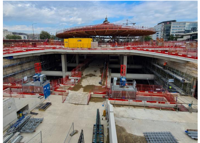
NCH site at RER A first basement level
