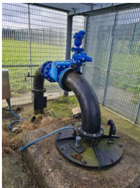
Typical borehole headworks Multi-stage borehole pump
