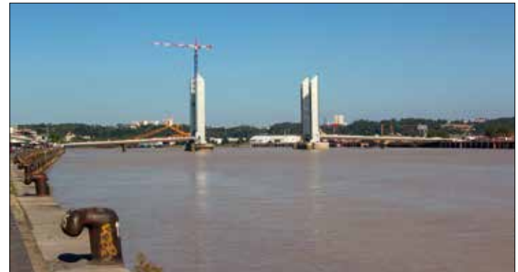
13.20 The Bacalan Bastide lifting bridge
