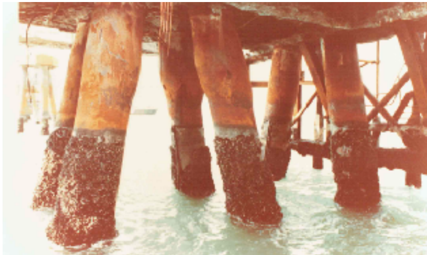
Damaged Piles
